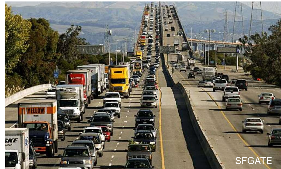
San Mateo Bridge West Bound
